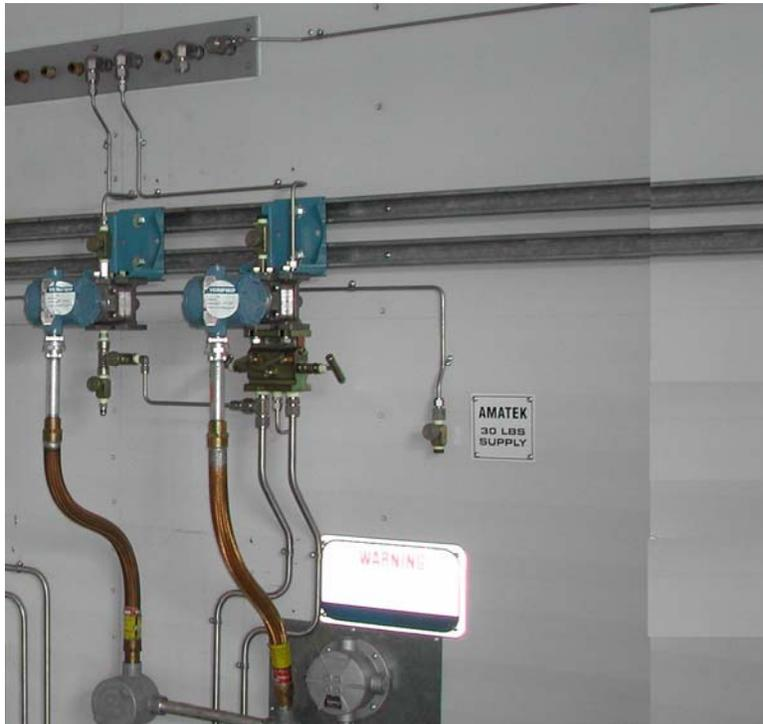
Then you add two more differential pressure transmitters, valves, tubing and wiring:
